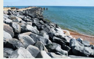
ROCK ARMOUR/RIP RAP
